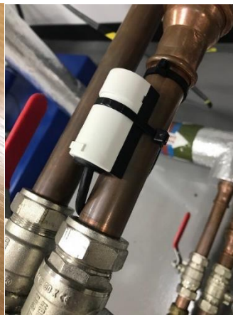
Flow Temperature Sensor on pipework
