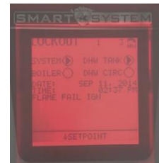
Boiler is not working
