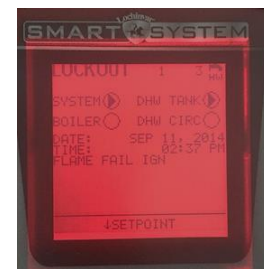
Boiler is not working
