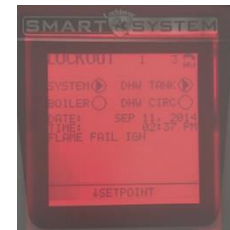
Water Heater is not working
