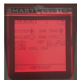
Water heater Locked out
