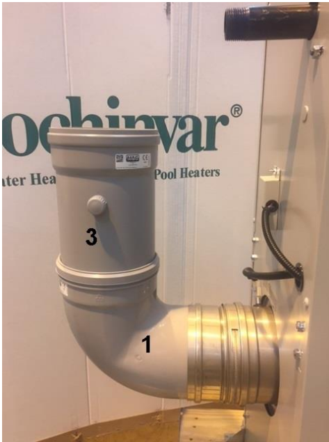
EXHAUST TRANSITION KIT FITTED EKW206CE-EKW236CE
