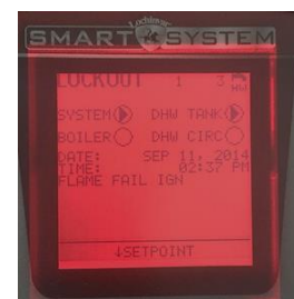
Water heater Locked out
