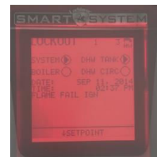
Water Heater is not working
