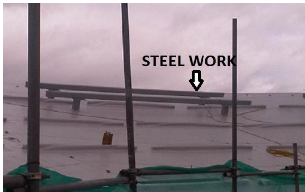
Steel work on roof
