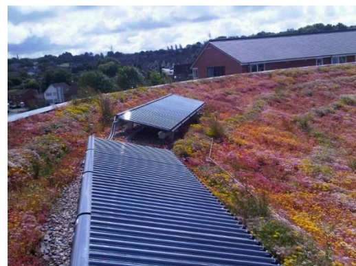
Collectors fitted to steel work
