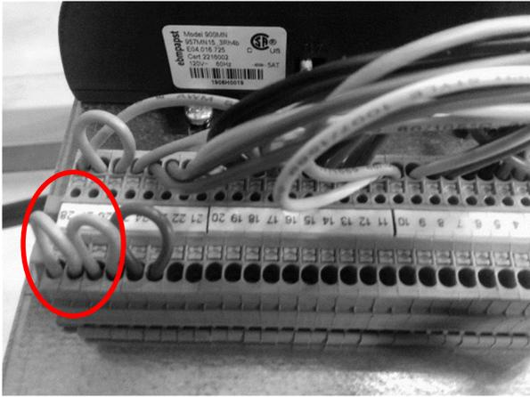
Low voltage connections EFB boiler.
