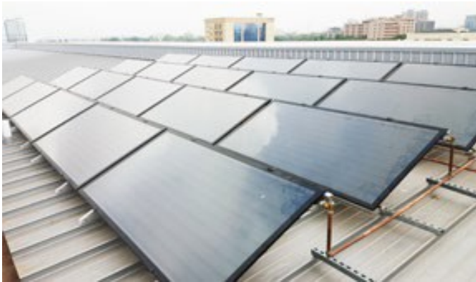
Metal roof with upstand
