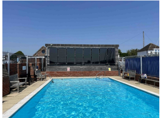
On roof frame vertical wall fixing
