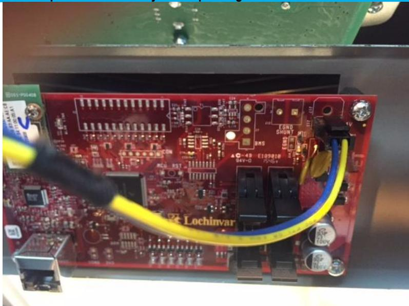
**16. Tidy all loose cables into the cable clamps fitted within the unit.**
