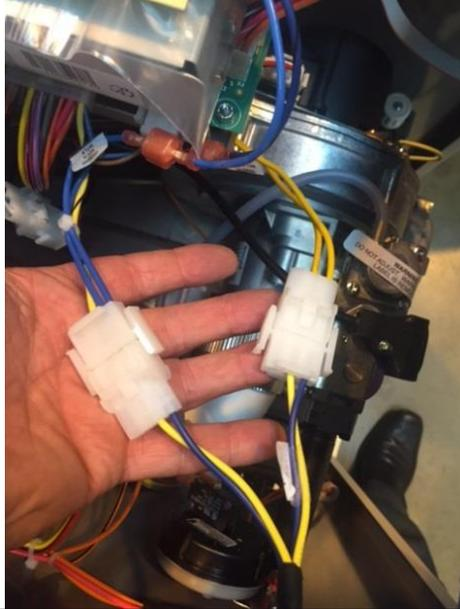
15. Fit the other end of the Con-X-us power harness to the Con-X-us board. Make sure the plug connector is positioned correctly before pushing onto the Con-X-us board.
