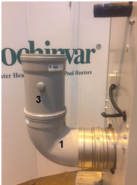
EXHAUST TRANSITION KIT FITTED EKW206CE-EKW236CE
