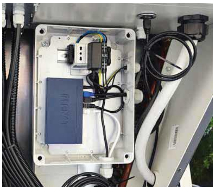
Cascade wiring centre showing ethernet connections
