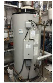
Typical pre-2019 installation
