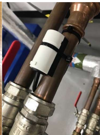
Flow Temperature Sensor on pipework
