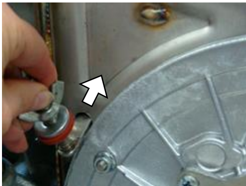
Position the plug into heat exchanger:
