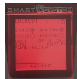
Boiler is not working
