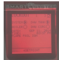
Boiler is not working
