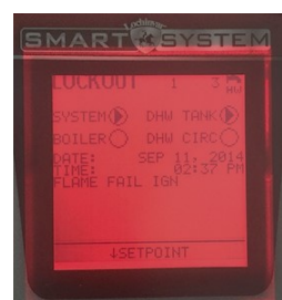
Boiler is not working
