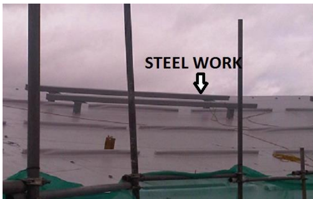
Steel work on roof
