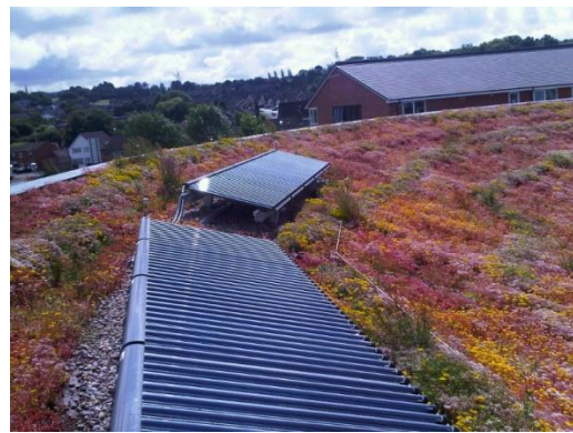
Collectors fitted to steel work
