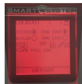
Water heater Locked out
